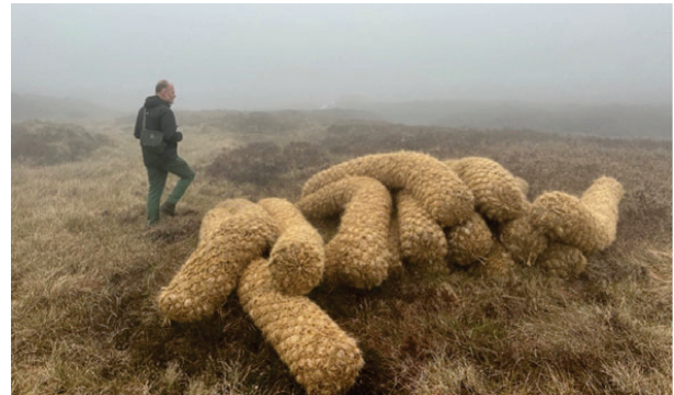
• Figure 4: Coir logs used in peatland restoration at Cuilcagh Anierin Uplands.
