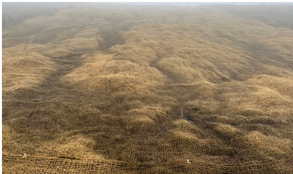
• Figure 3: Geotextile material used in peatland restoration at Cuilcagh Anierin Uplands.
