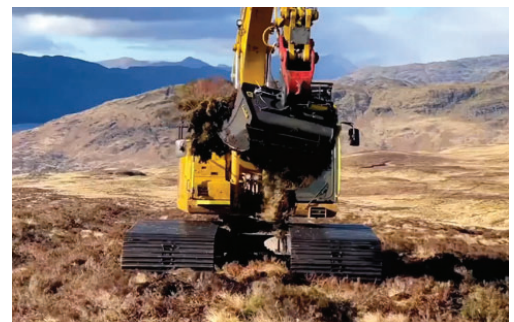
• Figure 15 and 16: Excavator working on site at Loch Katrine © Scottish Water.
