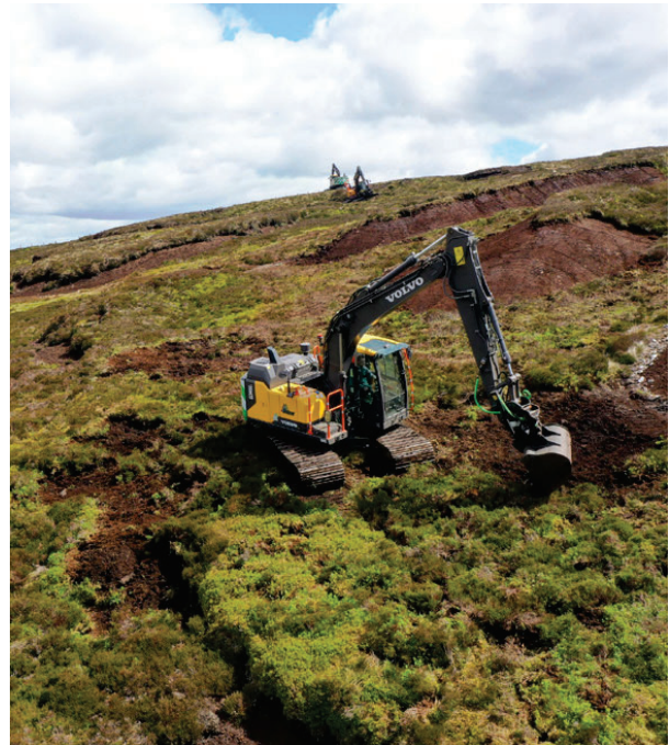
• Figure 12: Excavators at work in the Backwater Reservoir catchment © Scottish Water.
